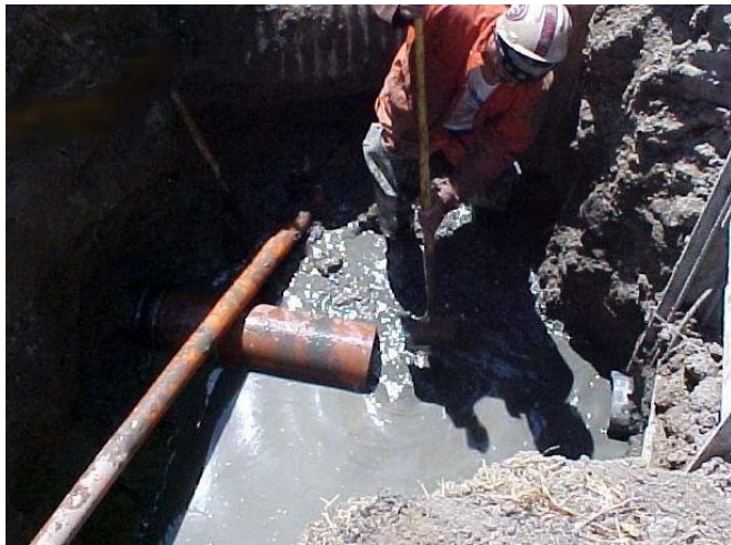
Worker repairs sewer main at Shepherd Canyon.
